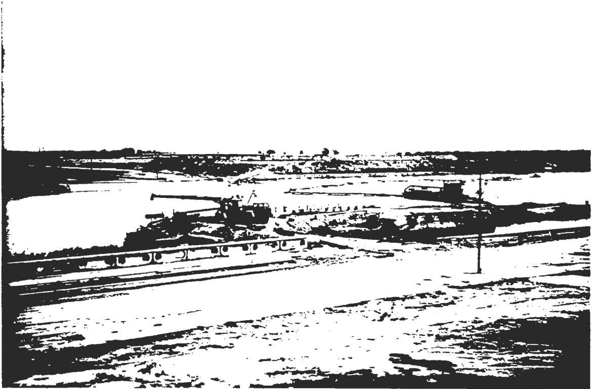
Figure 17.5. The Kara Kum Canal near the capital city of Ashgabat, with concrete sides being installed to limit water loss. Photo by P. P. Micklin.
