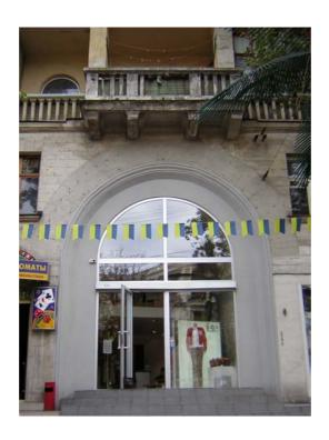
floor above. The balcony and the Doric-styled balustrade that serves as a railing are disintegrating. In one section of six balusters, five are missing, which leaves only the one baluster at the far right supporting the section. Much like "Megasport" the newly painted facade
