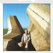
**The Dolos:** This unusually shaped concrete block weighs up to 20 tons, and is used to protect harbor walls from the force of the sea. Dolosse works by dissipating the energy of the waves, instead of blocking it. Dolosse was designed by harbor engineer Eric Merrifield, and was first installed in East London. Unfortunately, this breakwater device was never patented, and has been copied all over the world.
