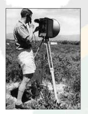
**Tellurometer:** Before 1955, land surveying depended on timeconsuming and complicated manual methods to measure distance. The world of map making was revolutionized when Trevor Wadley invented the Tellurometer, which was developed from radar techniques from World War II. This device is capable of measuring distances of up to 50km with an accuracy of millimeters.
